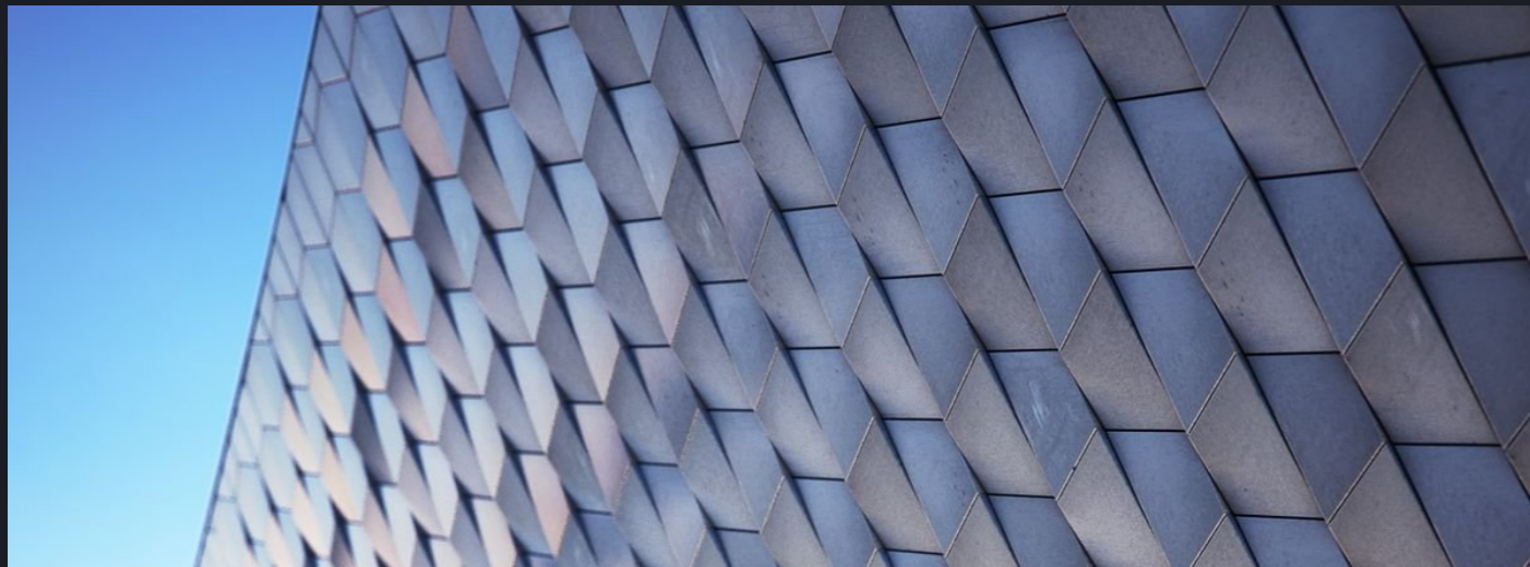
FIG. 3 — CURVED FAÇADE AT SCALE. THE CODE IS A COORDINATION INSTRUMENT, NOT A CLAUSE LIST.
